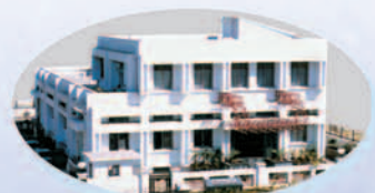
State Of The Art Manufacturing Plant at Navi Mumbai
